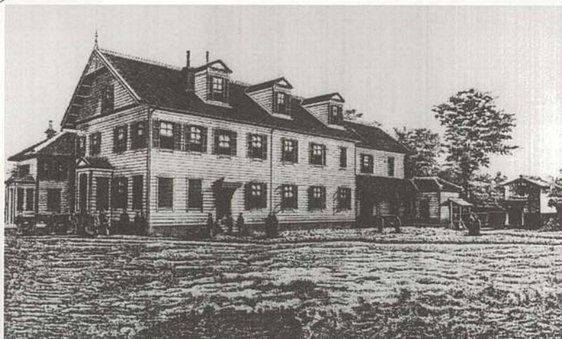
GIRLS SCHOOL BUILDING IN THE CITY OF SENDAI, MIYAGI KEN, JAPAN. The property of the Board of Commissioners for Foreign Missions of the Reformed Church in the United States. Dedicated July 5, 1889.
