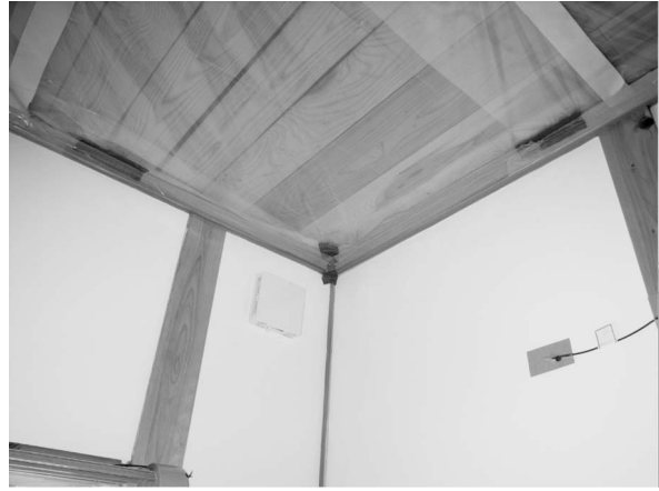
Figure 6. Sealing with Tape and sheet
